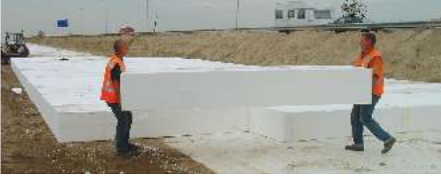
Photo Source: European Manufacturers of Expanded Polystyrene (EUMEPS) Master Class (2010). EPS in Civil Engineering Applications, November 16th & 17th, 2010, Amsterdam – the Netherlands
