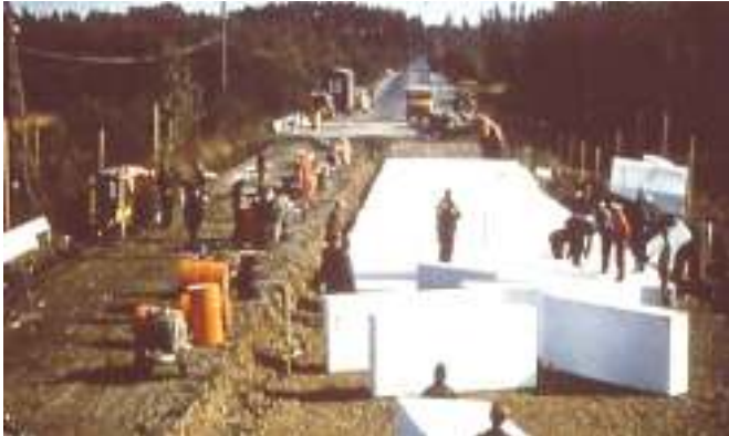
First EPS Block Application (Source: Alfheim, S., Flaate, K., Refsdal, G., Rygg, N., and Aarhus, K., 2011. The first EPS Geoblock Road Embankment - 1972, Proceedings of the 4th International Conference on Geofoam Blocks in Construction Applications, EPS 2011, Lillestrøm, Norway.)
