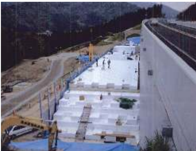
EPS Block Highway fill (Source: Aunaas, K. (2011) Recent impressions from EPS projects in Japan. Proceedings of the 4th International Conference on Geofoam Blocks in Construction Applications, EPS 2011, Lillestrøm, Norway.)
