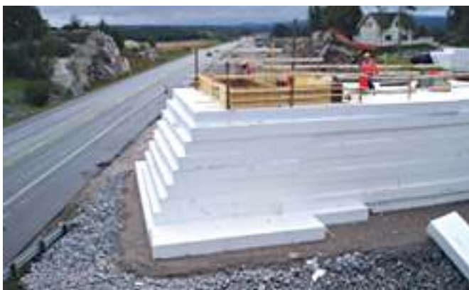
Grimsøyveien Bridge (Source: Damteu, T., Vaslestad, J. & Refsdal, G., 2011. Case histories with EPS geofoam embankments from eastern Norway. Proceedings of the 4th International Conference on Geofoam Blocks in Construction Applications, Lillestrøm, Norway).
