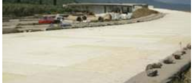
Production of EPS Block Bridge Approach fill (Source : Papacharalampous, G. and Sotiropoulos, E.,2011. First time application of expanded polystyrene in highway projects in Greece. Proceedings of the 4th International Conference on Geofoam Blocks in Construction Applications, EPS 2011, Lillestrøm, Norway.)
