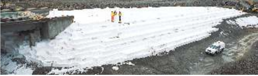
Photo Source: European Manufacturers of Expanded Polystyrene (EUMEPS) Master Class (2010). EPS in Civil Engineering Applications, November 16th & 17th, 2010, Amsterdam – the Netherlands.
