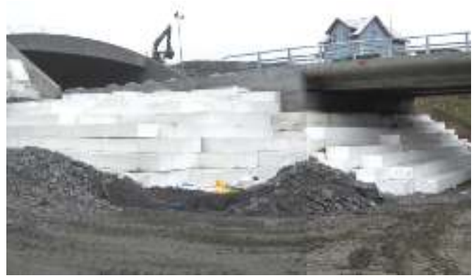
EPS Block bridge and culvert fills (Source: Damteu, T., Vaslestad, J., and Refsdal, G. (2011) Case histories with EPS geofoam embankments from eastern Norway. Proceedings of the 4th International Conference on Geofoam Blocks in Construction Applications, EPS 2011, Lillestrøm, Norway.)
