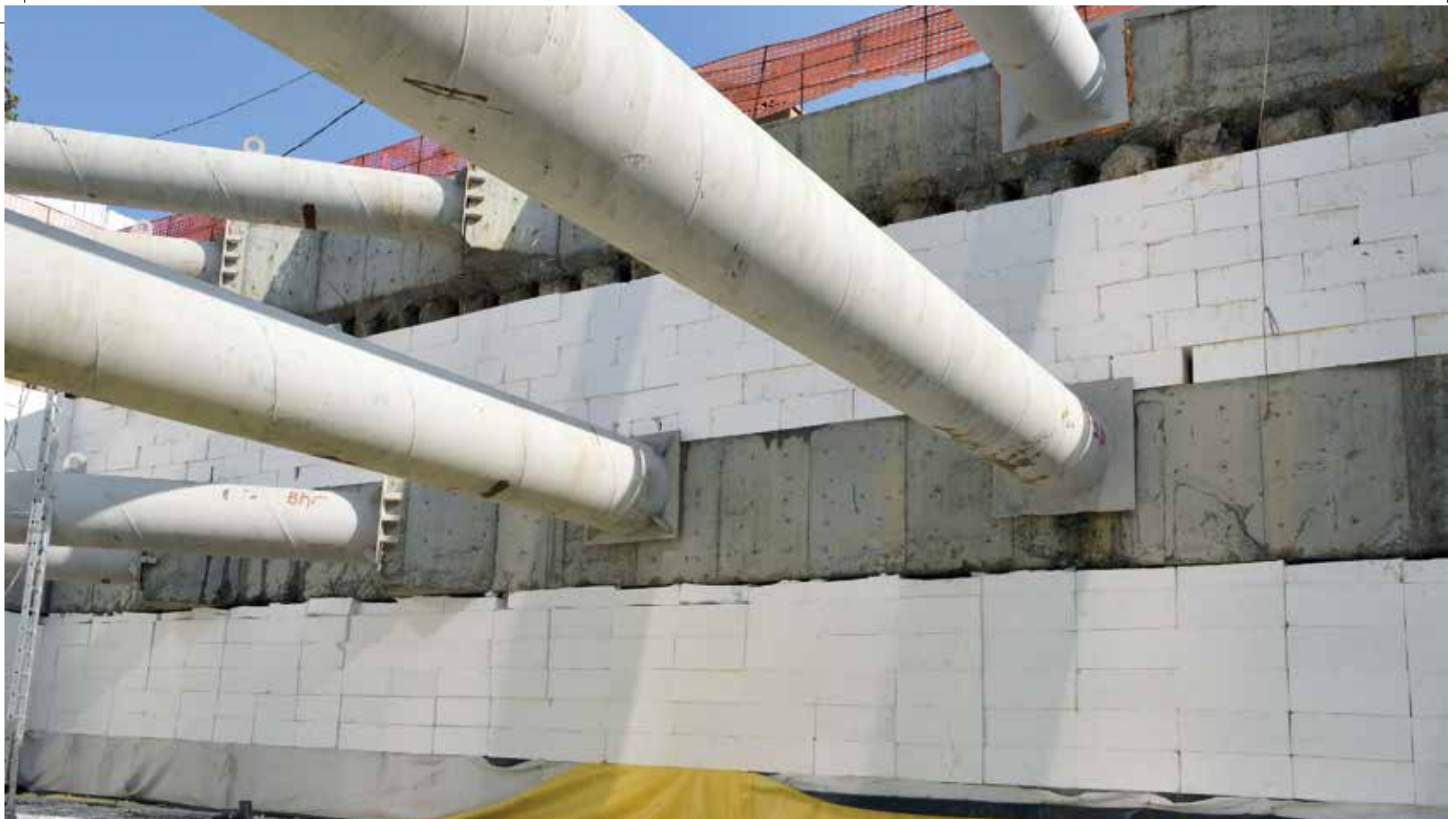
LIGHTWEIGHT FILL APPLICATION IN BETWEEN WALER BEAMS OF DRILLED SHAFTS
