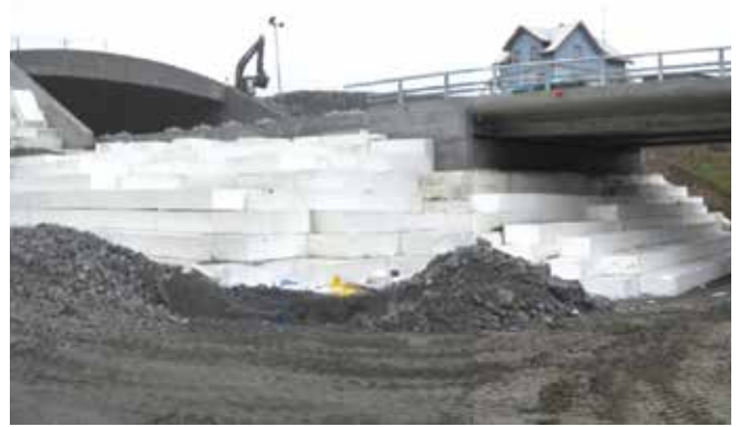
EPS Blok köprü ve menfez dolguları (Kaynak: Damteu, T., Vaslestad, J., and Refsdal, G. (2011) Case histories with EPS geofoam embankments from eastern Norway. Proceedings of the 4th International Conference on Geofoam Blocks in Construction Applications, EPS 2011, Lillestrøm, Norway.)
