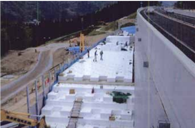
EPS Blok otoyol dolgusu (Kaynak: Aunaas, K. (2011) Recent impressions from EPS projects in Japan. Proceedings of the 4th International Conference on Geofoam Blocks in Construction Applications, EPS 2011, Lillestrøm, Norway.)
