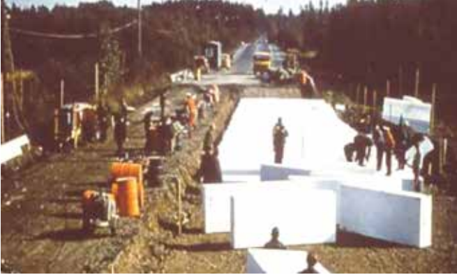
İlk EPS Blok Uygulaması (Kaynak: Alfheim, S., Flaate, K., Refsdal, G., Rygg, N., ve Aarhus, K., 2011. The first EPS Geoblock Road Embankment - 1972, Proceedings of the 4th International Conference on Geofoam Blocks in Construction Applications, EPS 2011, Lillestrøm, Norway.)
