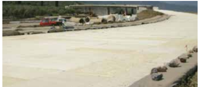
EPS Blok Köprü Yaklaşım Dolgusu İmalatı (Kaynak: Papacharalampous, G. and Sotiropoulos, E., 2011. First time application of expanded polystyrene in highway projects in Greece. Proceedings of the 4th International Conference on Geofoam Blocks in Construction Applications, EPS 2011, Lillestrøm, Norway.)
